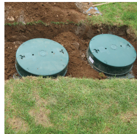
Tank risers ensure safety and accessibility for servicing.
