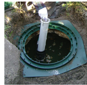
Homeowners can and should clean their effluent filters annually.
